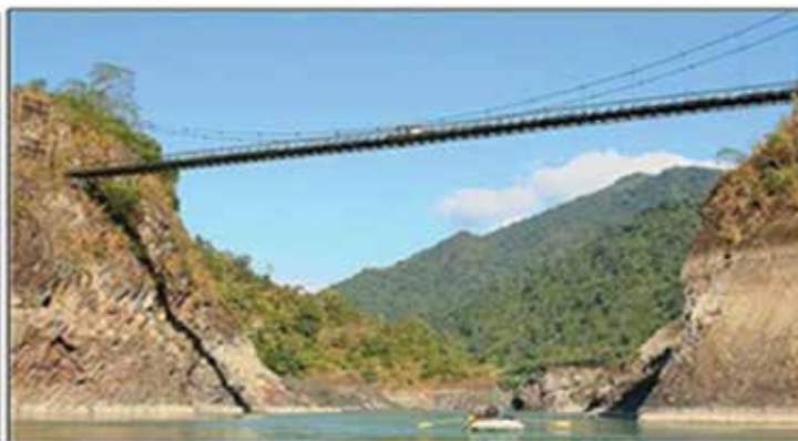
VIEW OF A 360 ft PRE-FAB SUSPENSION TYPE BRIDGE ON SIYOM RIVER, ARUNACHAL PRADESH, INDIA
